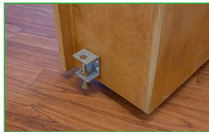
Outswing, support bolt bracket
